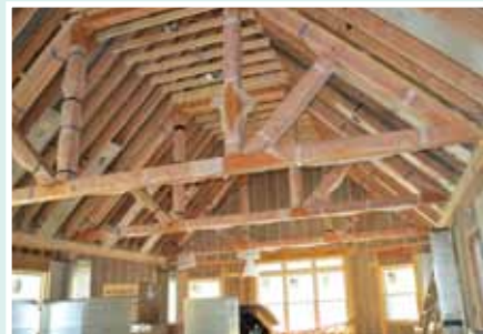
One of several sun-drenched and spacious workshop spaces in The Sarah Jane Herman Education and Resource Center.
